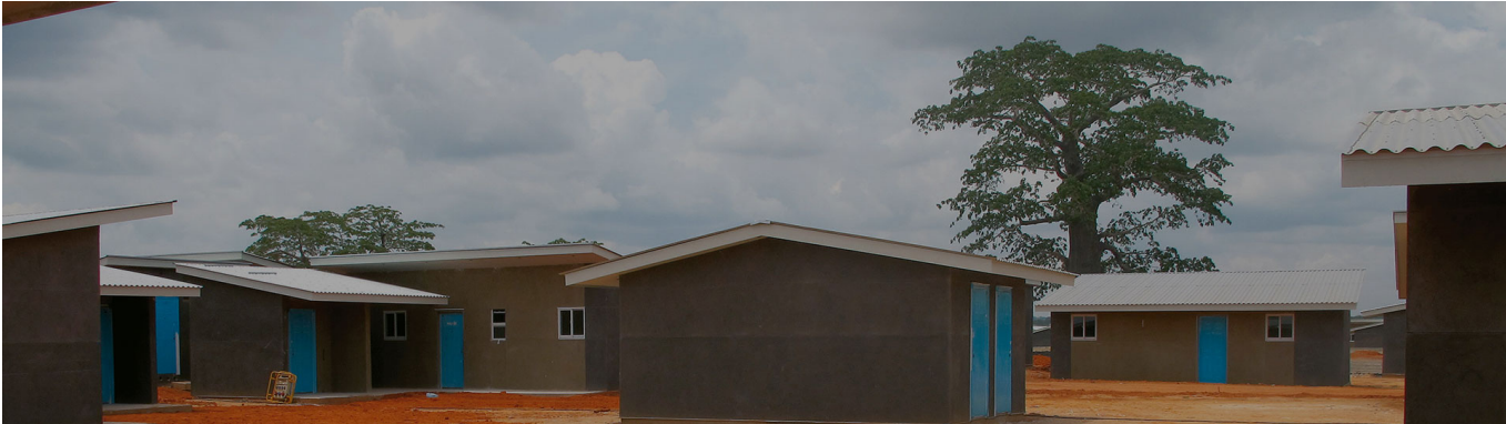
Aldeia Solar do Cabiri (Cabiri Solar Village)
