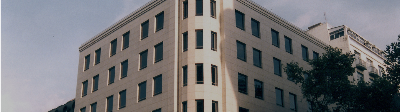
Deutsche Bank headquarters-building
